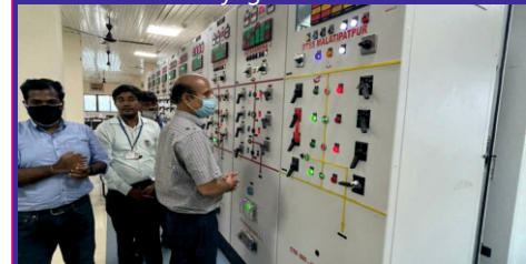
OPTCL commissioned 132 KVRTSS Malatipatpur line from Samagara ss on 25th June at 17:49 hrs.
