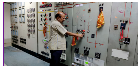
On 26th June OPTCL commissioned another railway traction transmission project at Bhalumaska in Rayagada district at 6:40 PM
